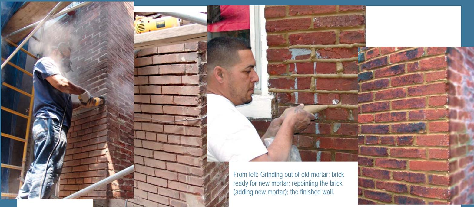
From left: Grinding out of old mortar; brick ready for new mortar; repointing the brick (adding new mortar); the finished wall.
