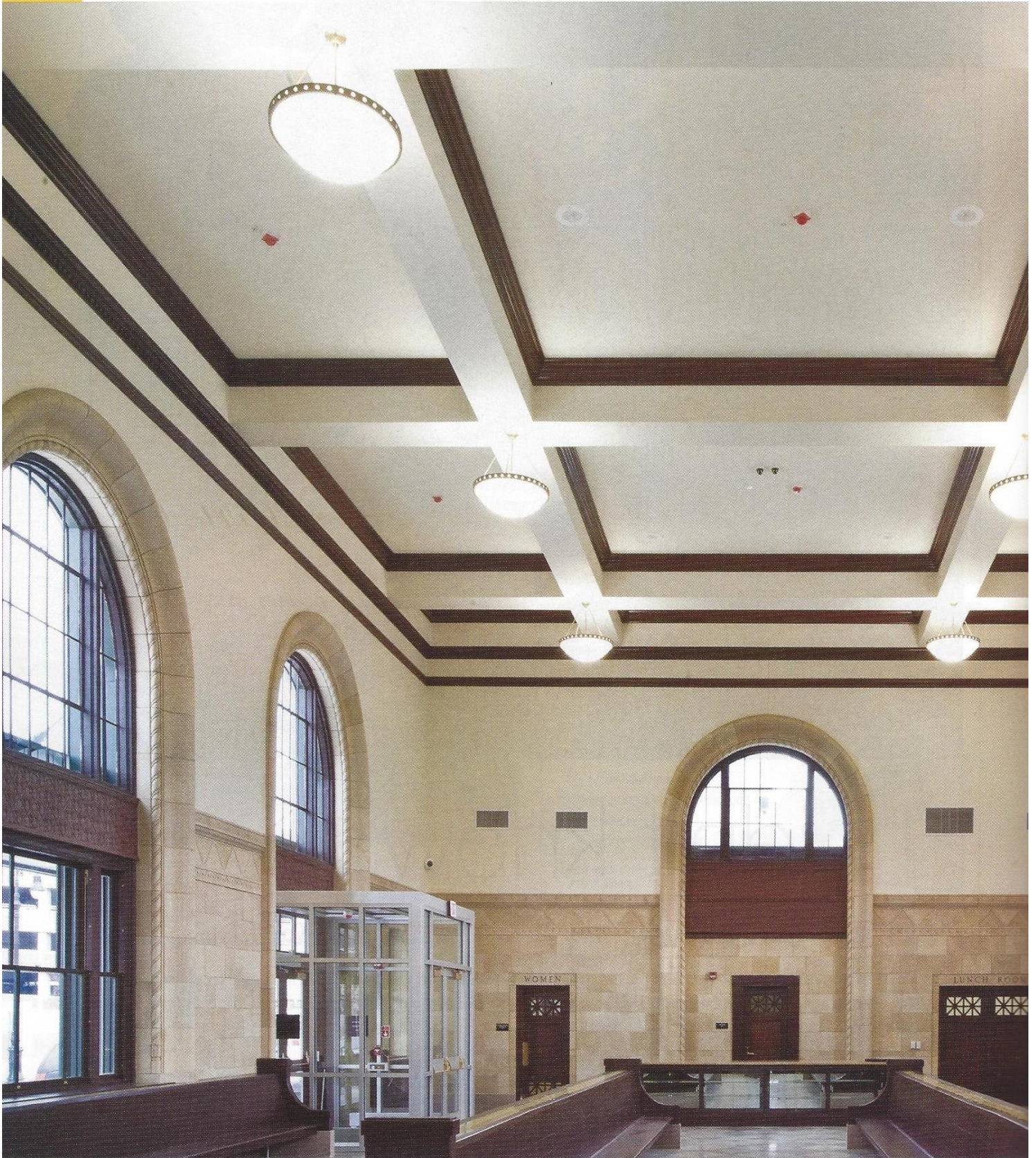
The beautifully restored coffered ceiling presented a millwork challenge.
